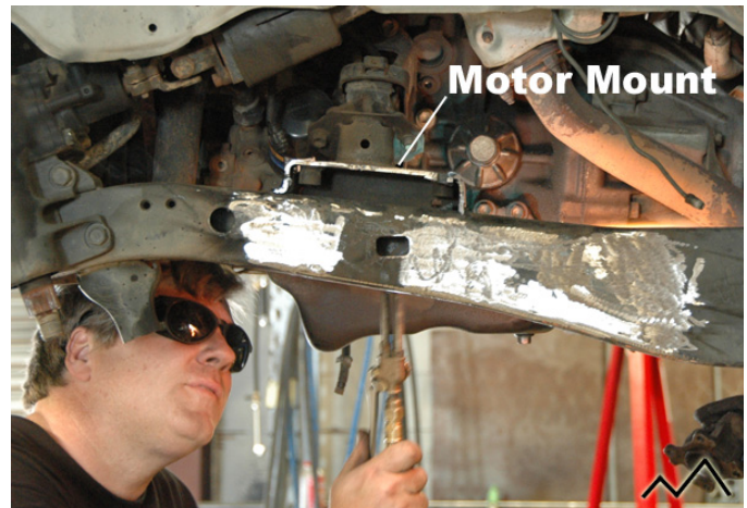
IFS Brackets Ground Off
