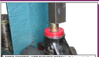
LOWER CONTROL ARM BUSHING INSTALL: Make sure inside surfaces are free of all old bushing material and sharp edges. Coat urethane bushing, sleeve and I.D. of lower control arm with supplied grease, all surfaces of bushings that contact metal. Press in bushing, hen press in sleeve.
