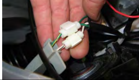
Indicator lamp wiring
