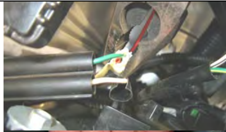
Running lamp wiring
