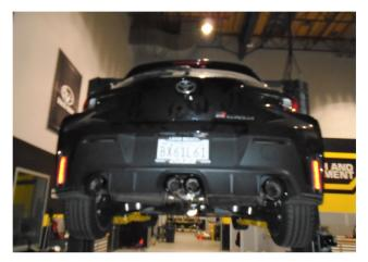
**Step 6:** Once a final position has been chosen for the new exhaust system, evenly tighten all clamps from front to rear using the torque specifications on page one of the instructions. Inspect all fasteners after 25-50 miles of operation and re-tighten if necessary.
